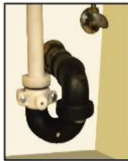
Drain pipe, p-trap and drain saddle
